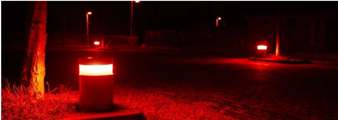
Figure 4: Example of low level bollard lighting
