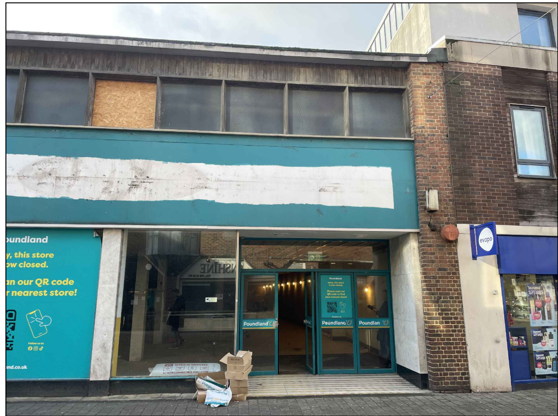
Photograph #2 Existing Front Elevation - RHS
