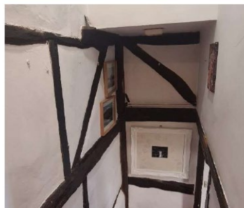
14) Rear original lower outshot area with crooked truss supporting the catslide; Original inglenook as part of once external end chimney; Original down braces in the northwest corner above modern staircase
