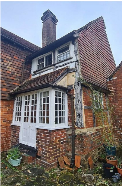
9) Two-storey south extension traditionally built in timber frame and originally infilled with brick. The porch was added later.
