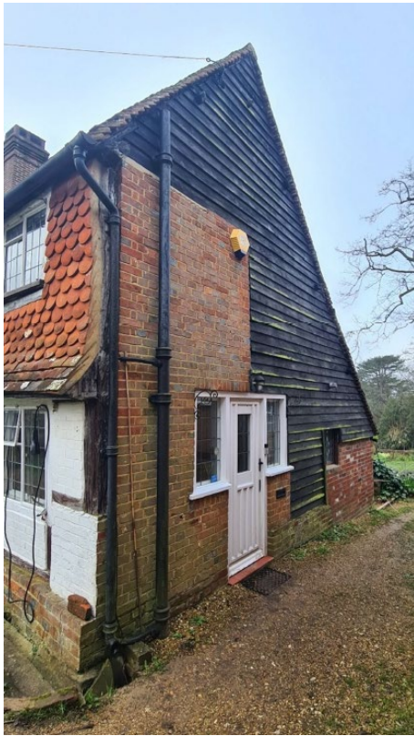
15) North facade weatherboarded and partially rebuilt in brick where earlier added external chimney was; South façade extended in timber frame and brick infill with Interwar porch added to the north side
