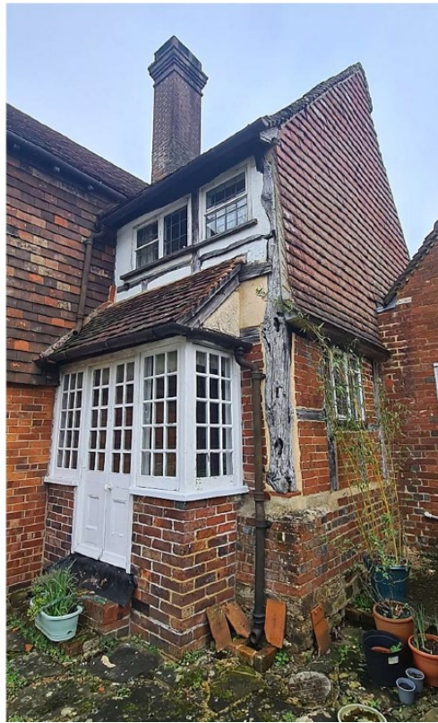
15) North facade weatherboarded and partially rebuilt in brick where earlier added external chimney was; South façade extended in timber frame and brick infill with Interwar porch added to the north side
