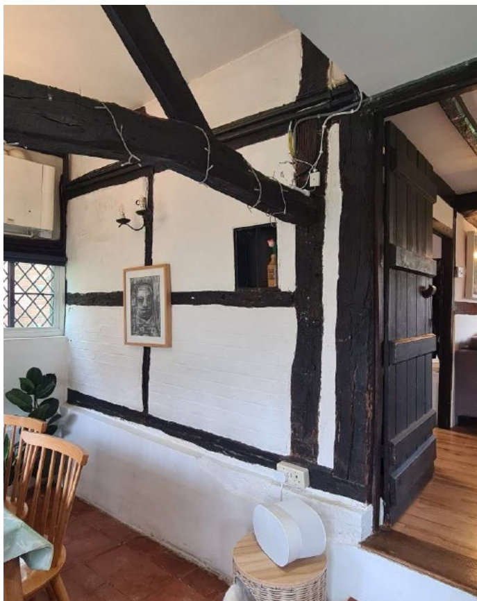
14) Rear original lower outshot area with crooked truss supporting the catslide; Original inglenook as part of once external end chimney; Original down braces in the northwest corner above modern staircase
