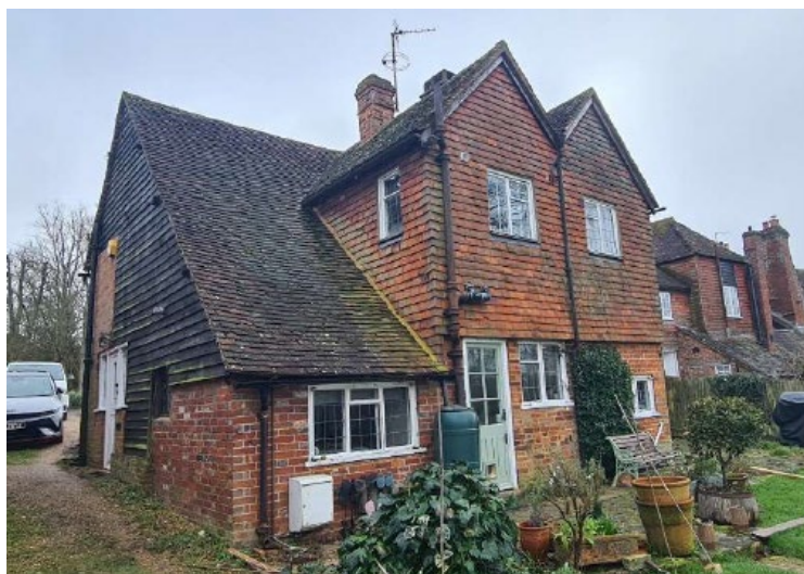
11) Rear extension today as it was built in the Late 1960s
