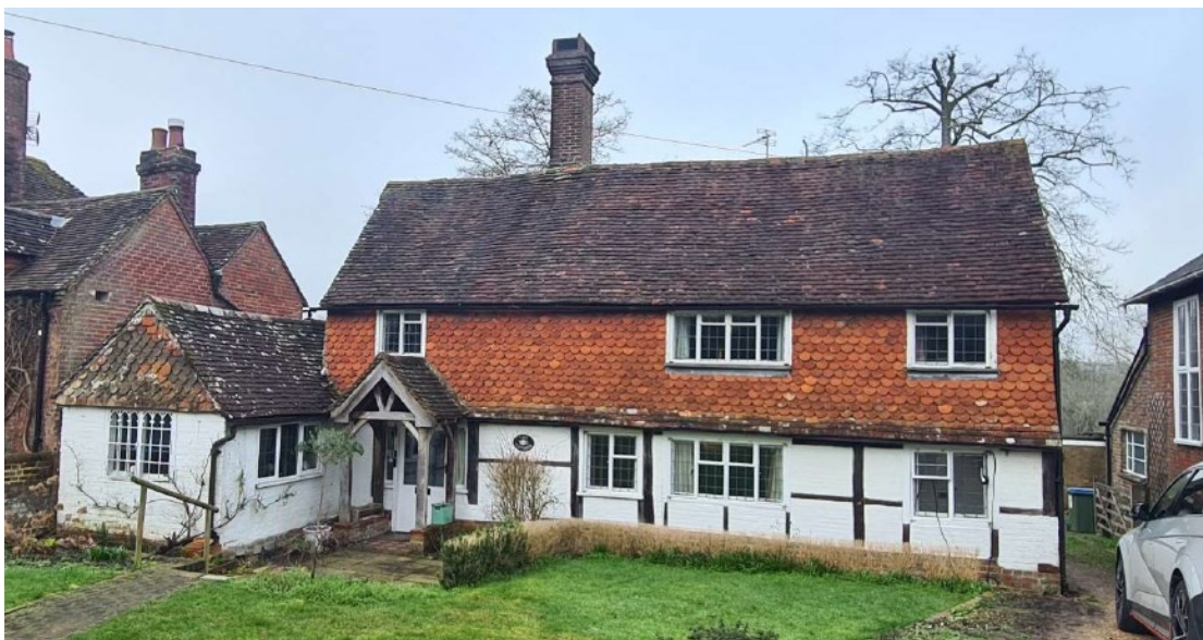
12) Front east facade at present with lower brick-infilled timber frame and upper tile-hung elevations
