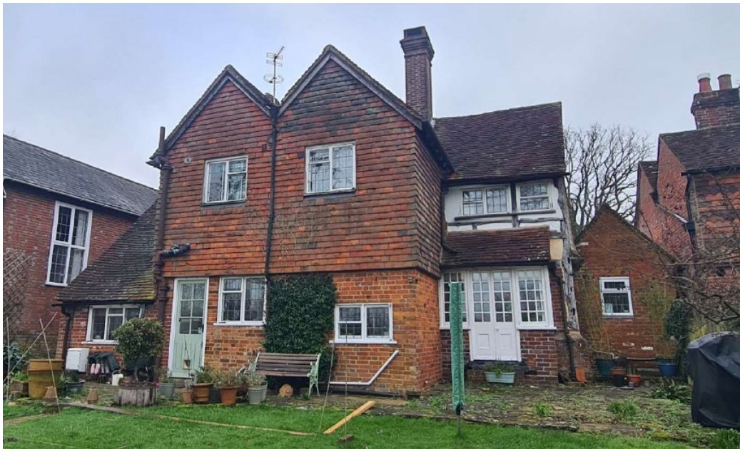
13) Rear west facade with catslide outshot, central 1960s two-storey extension, and south earlier extensions at present day
