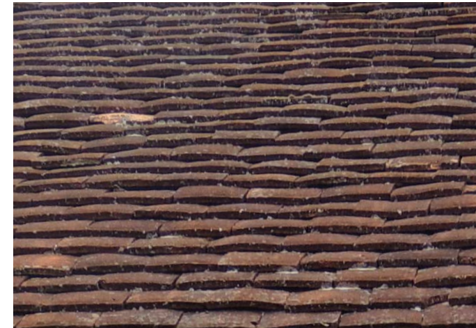
Plain clay roof tiles to match existing
