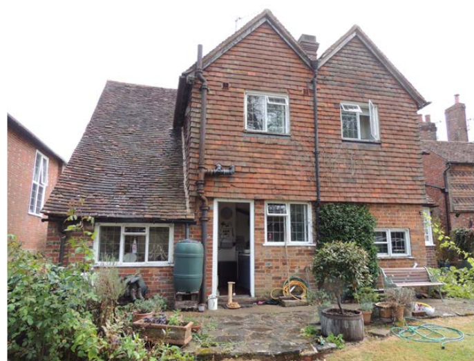
View of West Elevation
