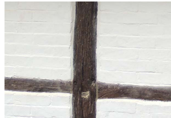
White painted brickwork and timber wall framing
