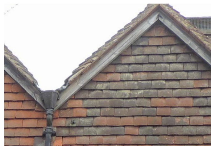
Timber fascias and cast iron rainwater goods
