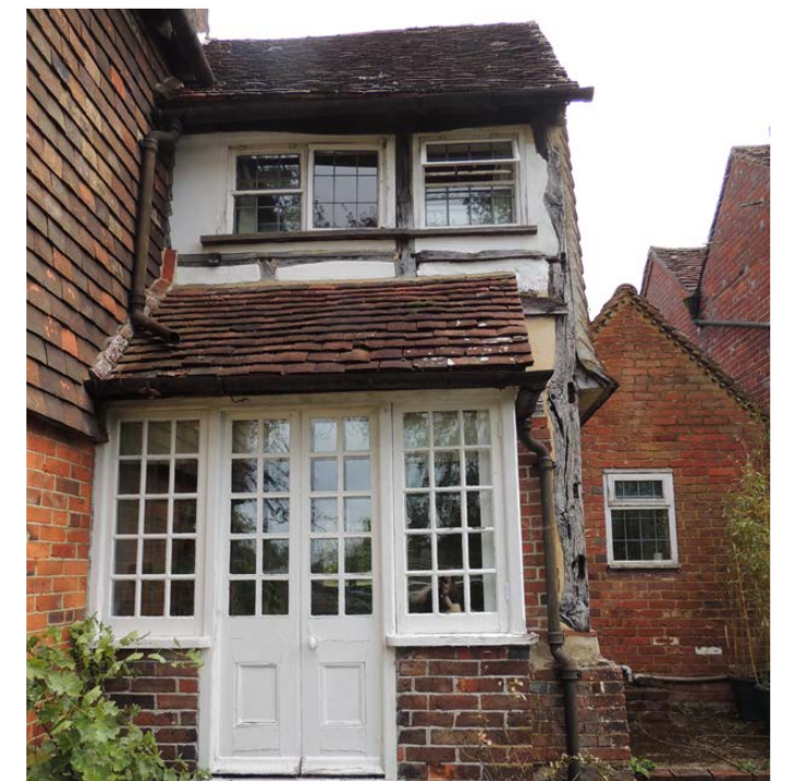
View of West Elevation
