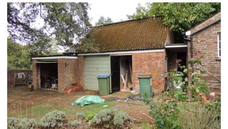
View of Garage
