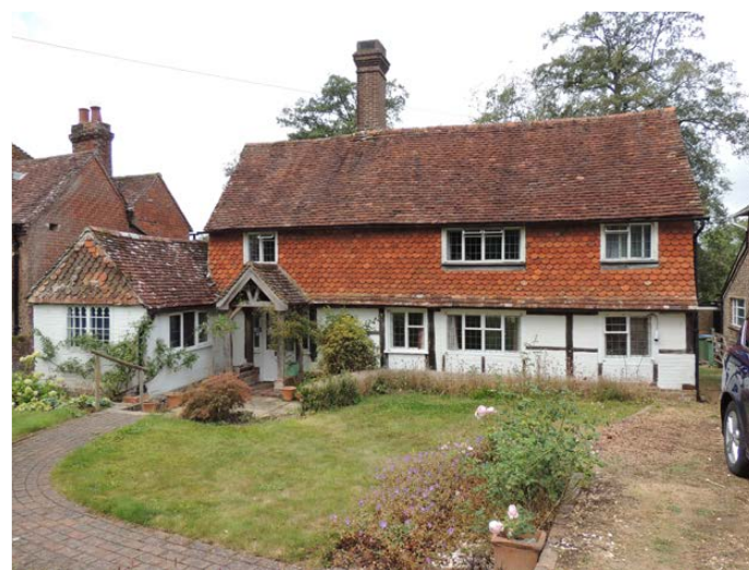
View of East Elevation
