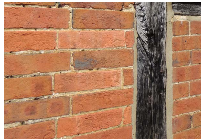
Unpainted red brickwork and timber wall framing
