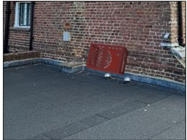
Flat Roof west side (above kitchen)
