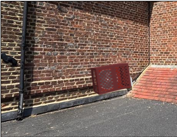
Flat Roof east side (above reception room)
