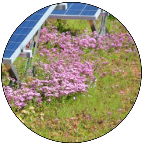
BIO-SOLAR GREEN ROOF (SEEDED)
