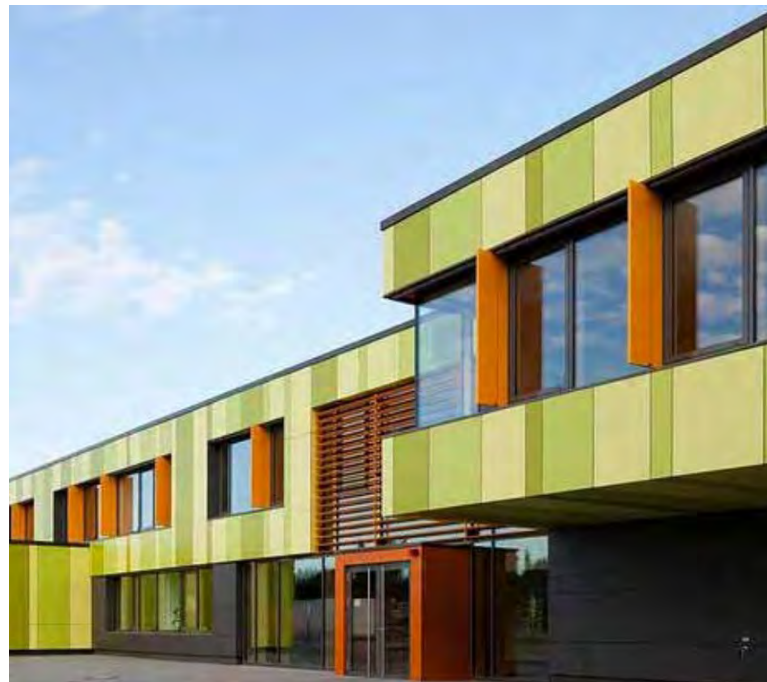
Consented scheme: Fibre cement cladding
