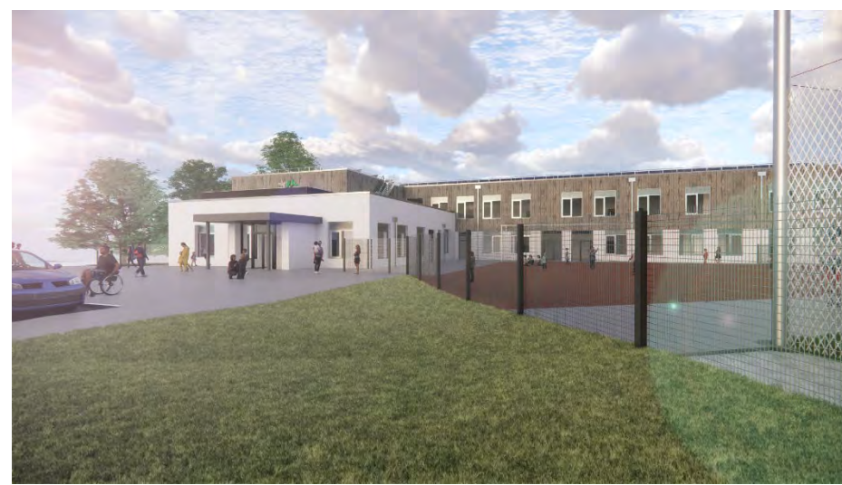
White brick and timber or 'cedral' clad first floor
