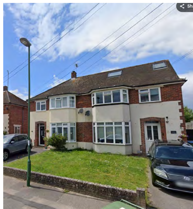
Mid century brick & render houses in Farm Ave.
