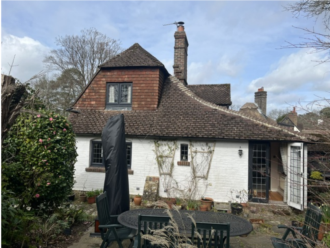
Existing south elevation – there appears to be an extension at the rear with a very shallow pitch.
