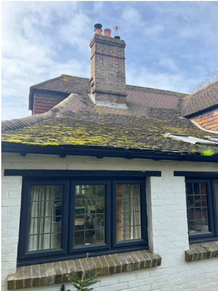
Existing east elevation – this shows the shallow pitched roof from the rear.
