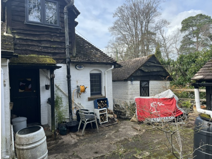
Existing east elevation – this shows the rear of the garage.
