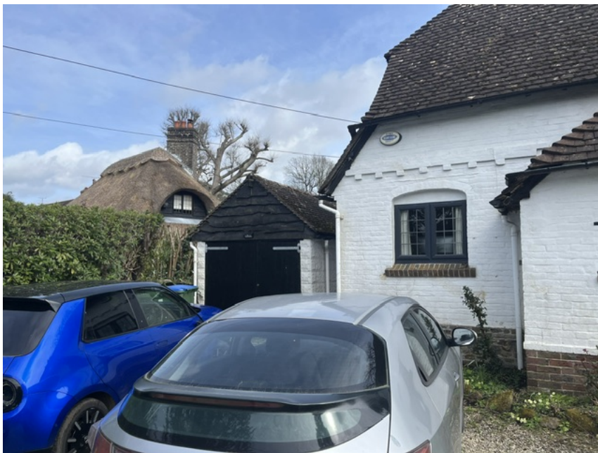
Existing east elevation – showing the garage
