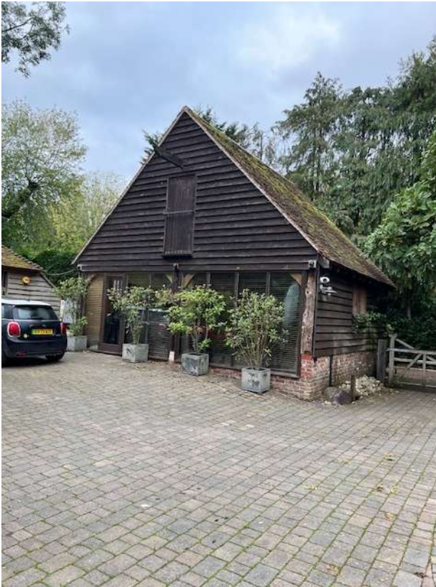
The Coach House Barn - East Elevation
