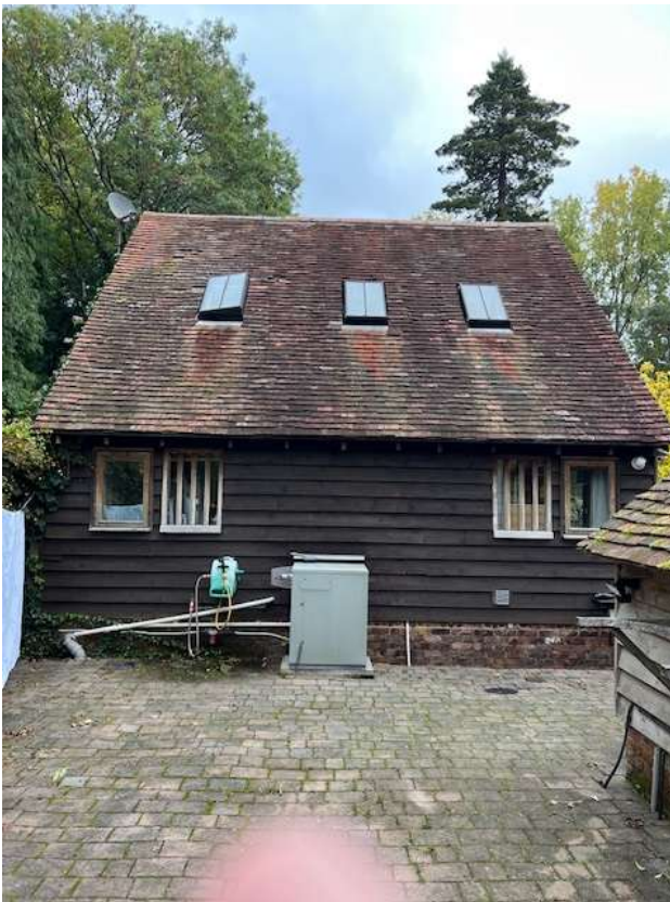
The Coach House Barn -South Elevation
