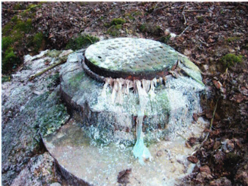
Pollution Flowing into Parsons Brook
