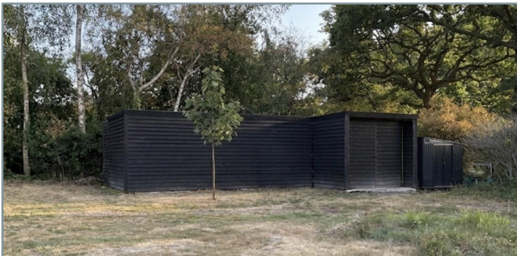
Above: Photo of existing storage building to be retained.
