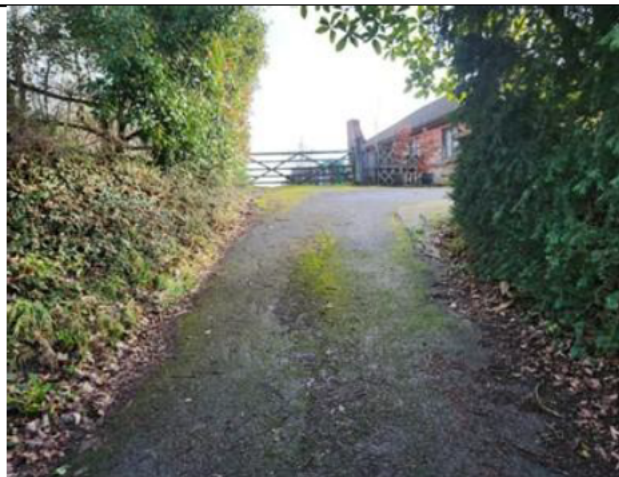
Photograph 10 – Tarmac access drive.
