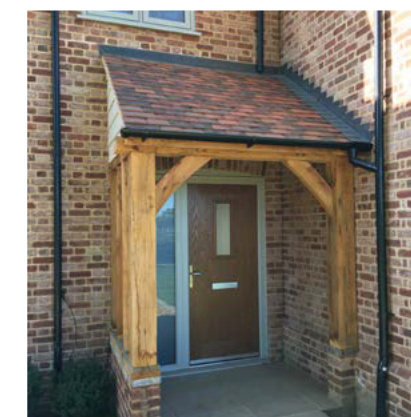
Lean to Porch with Timber Posts
