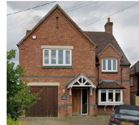
5. A281, 2 storey, red brick
