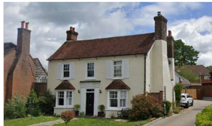
10. A281, 2 storey, painted brick
