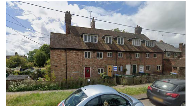
12. Station Road, 2 storey, multi brick
