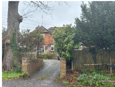
Properties in Henfield Road
