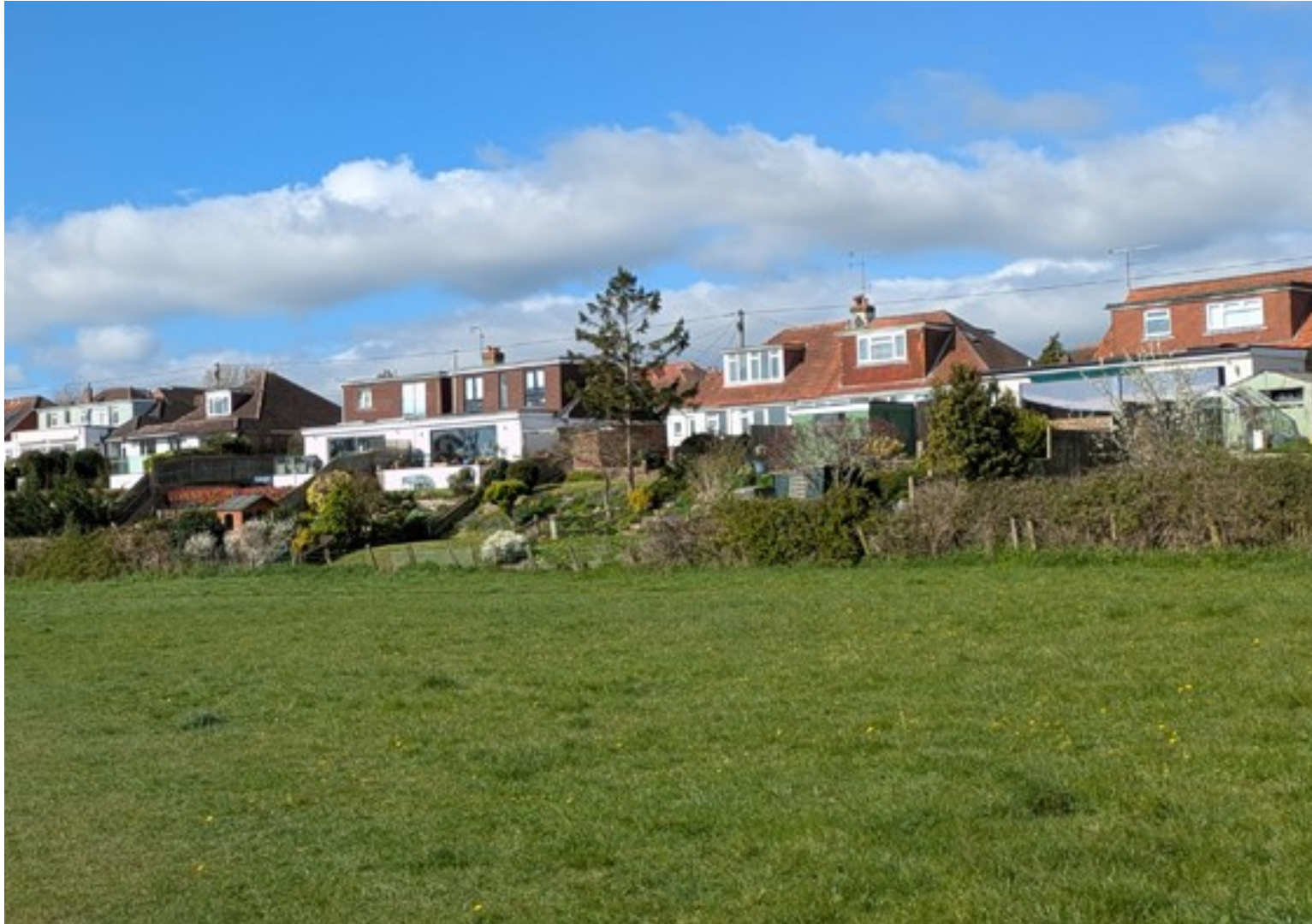
Rear elevation to Kings Stone Avenue immediately to SOUTH of number 37 showing varied roof extensions
