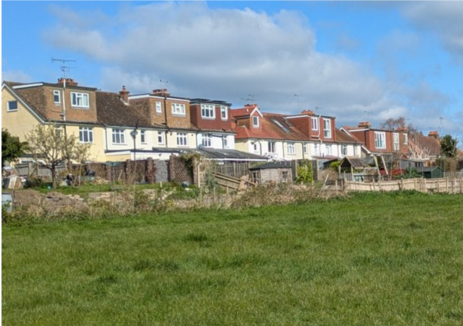
Rear elevation to Kings Stone Avenue immediately to NORTH of number 37 showing varied roof extensions
