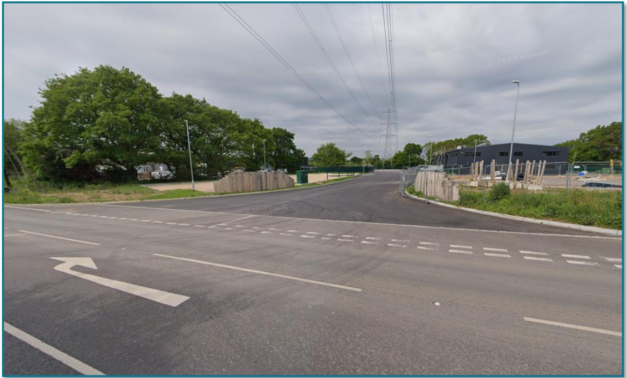
Figure 2.1 Access into the site with ghost right turn lane (built under approved application 'DC/20/0049')
