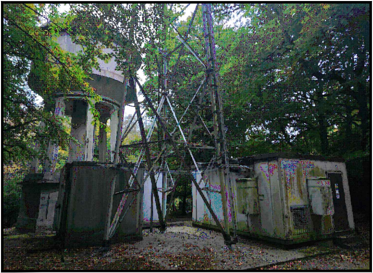
PHOTOGRAPH OF EXISTING SITE
