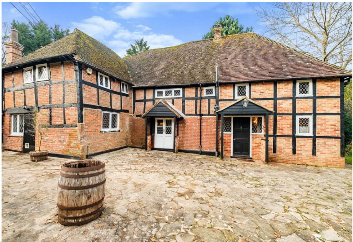
Fig 10: The 16 th Century dwelling of Blocques sits to the east of the site and is well set back from the highway. What awareness there is extends to glimpsed views when entering and exiting its curtilage.
