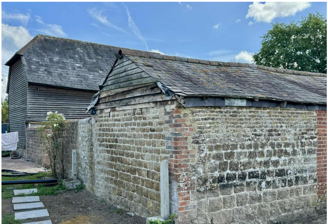
Fig 6: Sweetmans Barn forms part of a historic range of outbuildings to the western side of the site, enclosing a walled courtyard. The proposals would not result in any loss of historic fabric.
