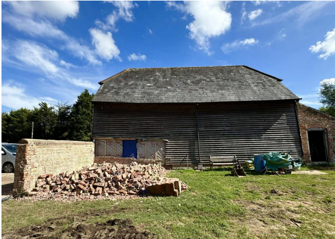
Fig 5: Sweetmans Barn comprises a former tithe barn, constructed from a timber frame with full height central door openings. Due to its age, it is considered to be a Non-Designated Heritage Asset.
