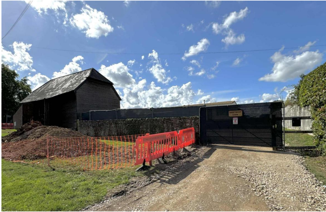
Fig 3: Sweetmans Barn dates from the 17 th Century and its principal elevation faces westwards, with its back to the highway. The proposed site makes a positive contribution to the setting of the listed buildings. © Chilcroft 2025
