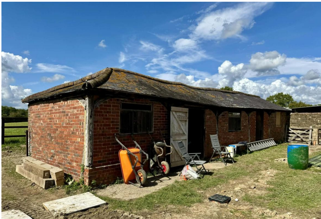
Fig 8: A single storey outbuildings sits to the rear of the proposed site and dates from the 18 th Century, being of a timber frame construction with stone walls to one end. Brick infill was added in the 20 th Century.
