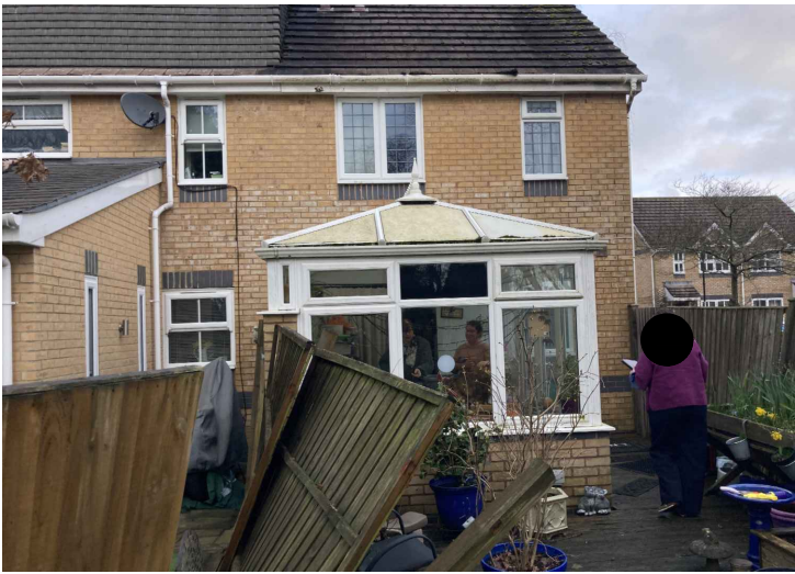
Photo 2: Existing rear elevation
