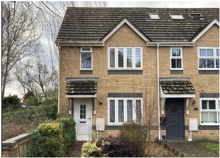
Photo 1: Existing front elevation
