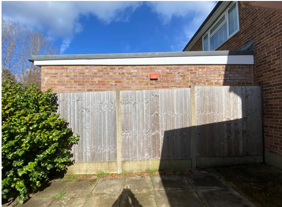
Side view of 6m wide rear extension at 49 Cootes Avenue
