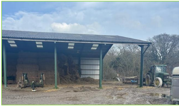
Two easterly bays. Viewed from the south.
