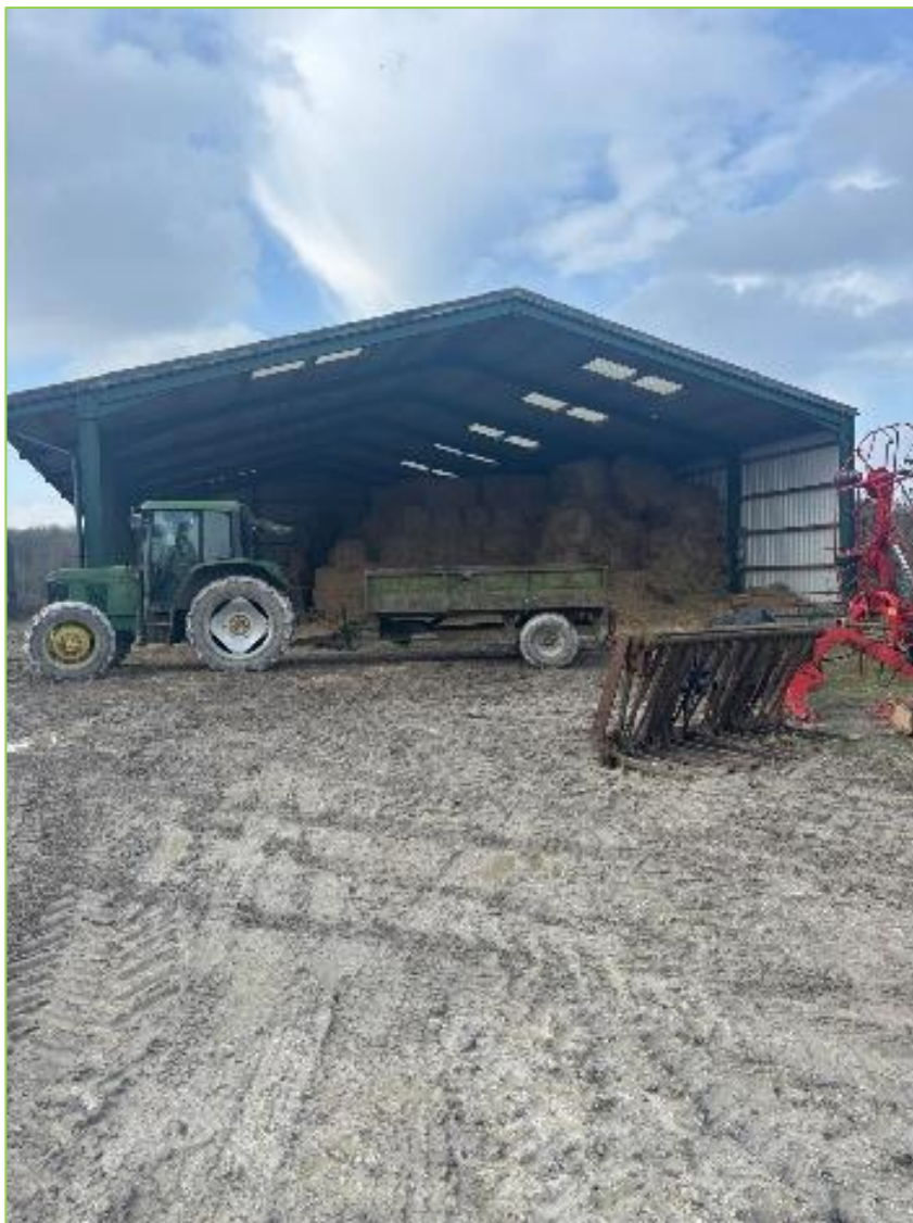
Hard-standing and eastern gable end of the building.
