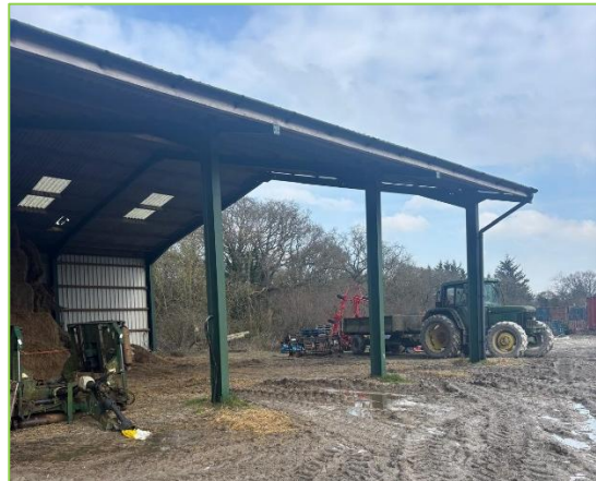
Two easterly bays. Viewed from the southwest.
