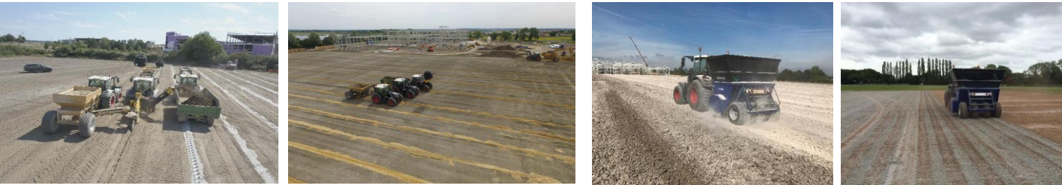
LAND DRAINAGE INSTALLATION AND SOIL AMELIORATION PROCESS
