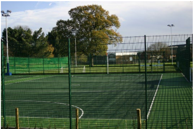
Porous Macadam Surface with textured paint application to achieve required slip resistance value (SRV) for both Netball and Tennis
