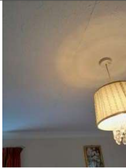
Minor hairline cracking from the wall up and across the ceiling in the bedroom in the extension.
