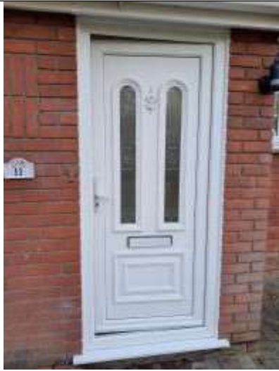
No separation or cracking to the brickwork around the door
