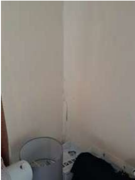
Minor separation in the extension bedroom where the wall joins the main building.
