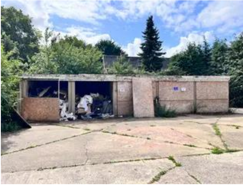
Photograph 6. The northern elevation of Building 4.
