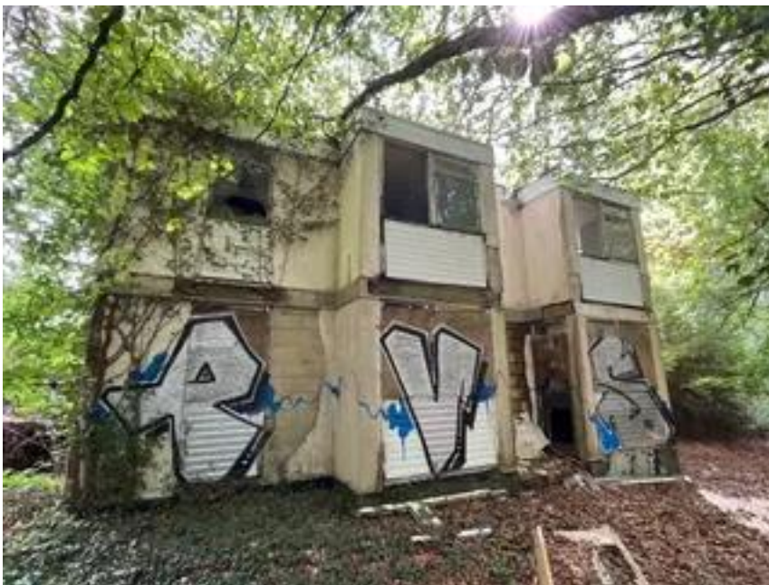
Photograph 9. The western elevation of Building 7.
