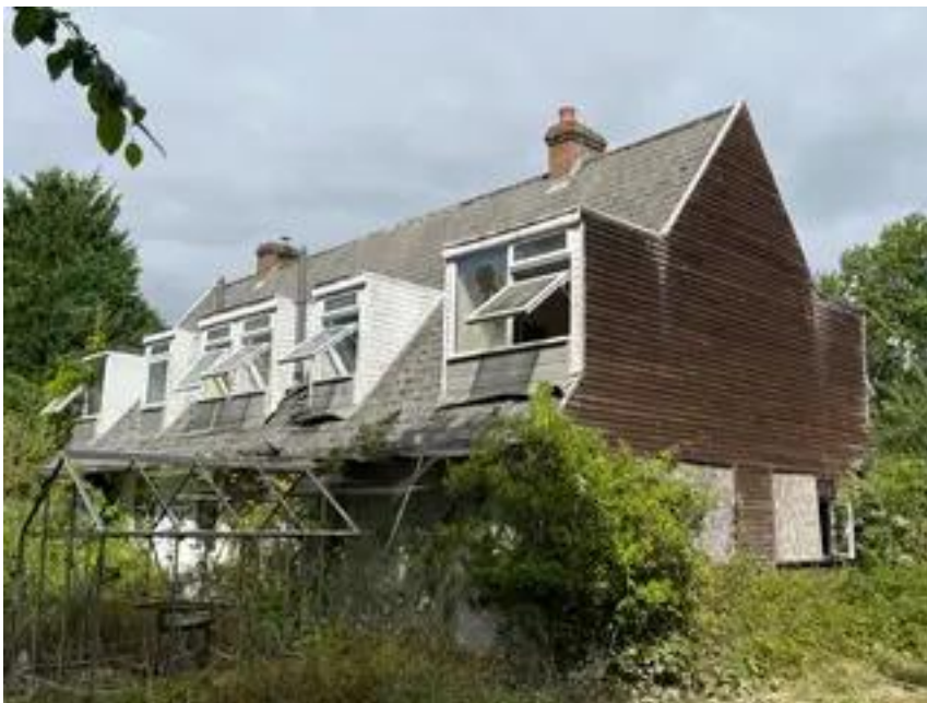
Photograph 7. The southern elevation of Building 5.
