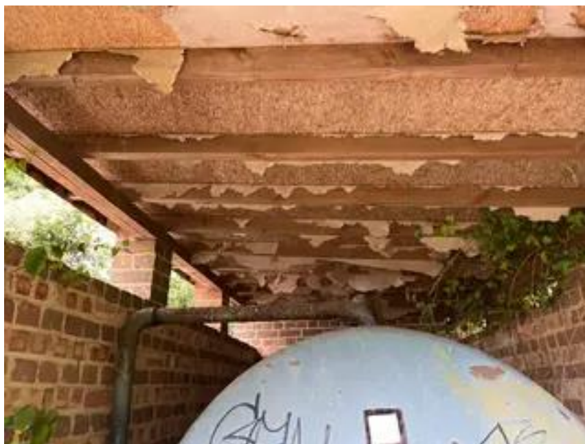
Photograph 4. The internal aspect of Building 3.
