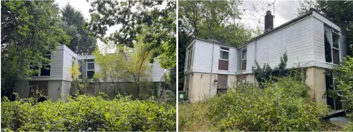
Photograph 10 & 11. Building 8 on the left and Building 9 on the right.
