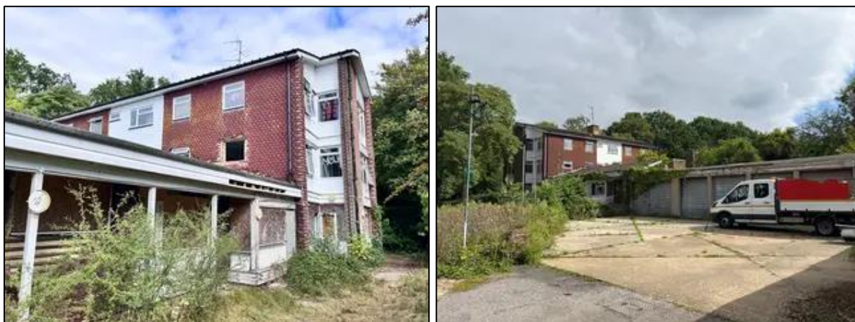
Photograph 1 & 2. The southern elevation of Building 1.
