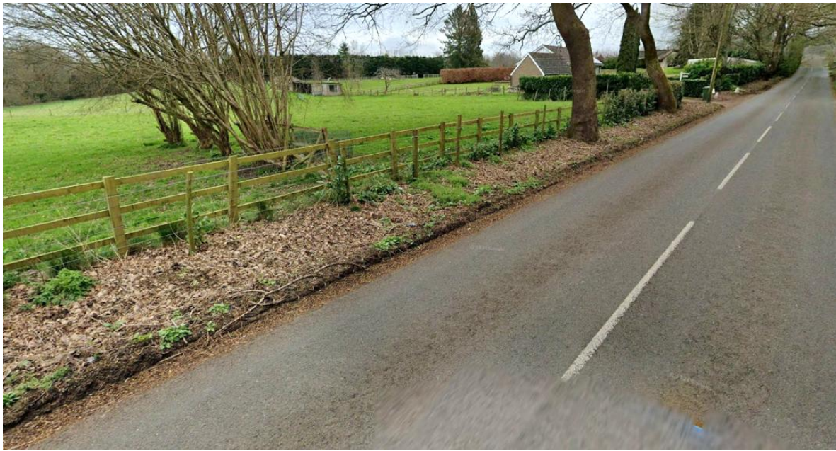
South splay from proposed new access point showing straight alignment of the road
