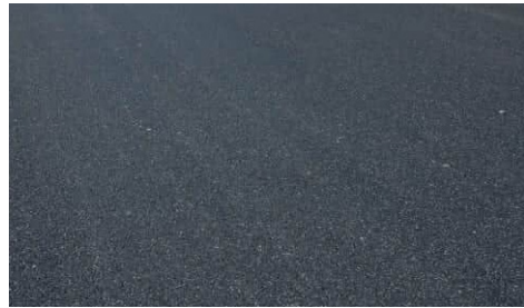
Heavy duty Asphalt - to primary access
