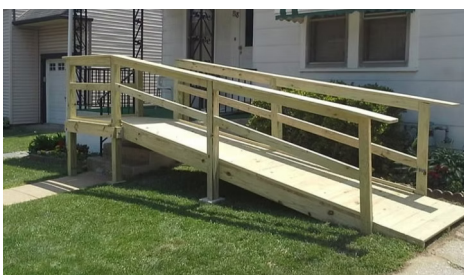
Timber Ramp - South-East School Building Access
