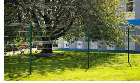
Euroguard Fencing - Surrounding Parts Of Phases 1 And 2 - 1.8m height
