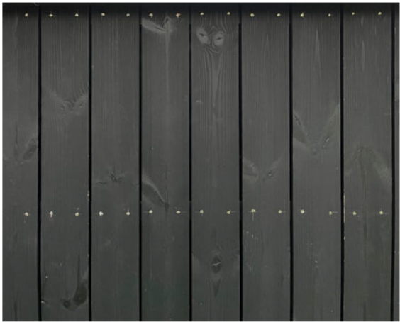
Dark stained timber external wall cladding
