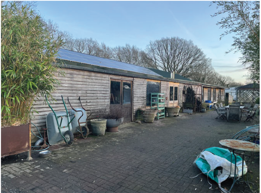
View towards south-west elevation
