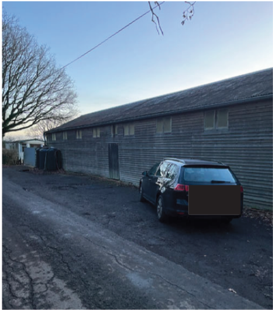
View of north-east elevation from lane
