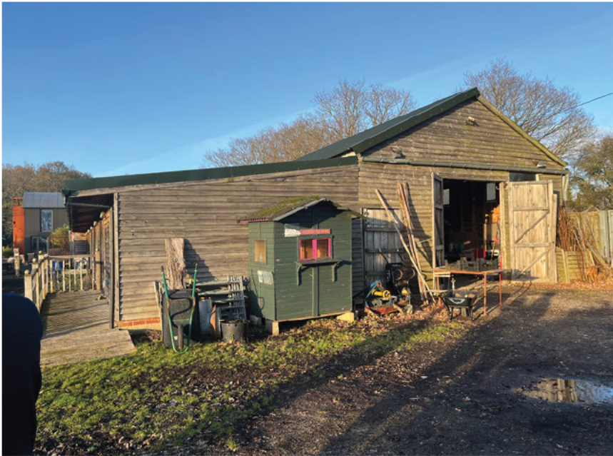
View of south east gable end
