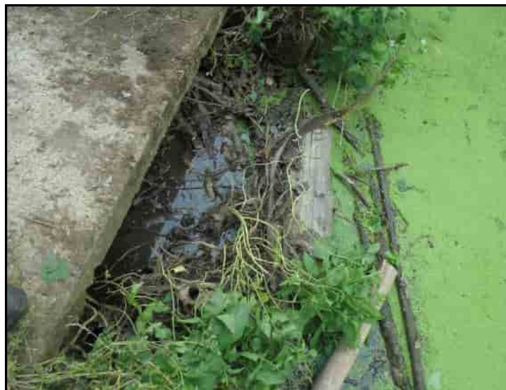
OF2 INTO SLABBED CHAMBER
