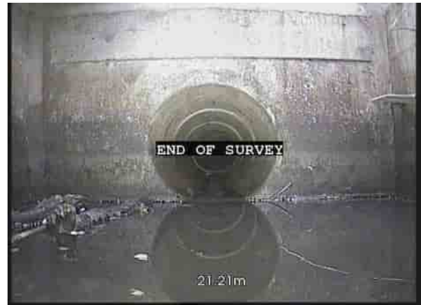
2, 00:01:43, 21.21 m Finish node, manhole, reference: IC1
