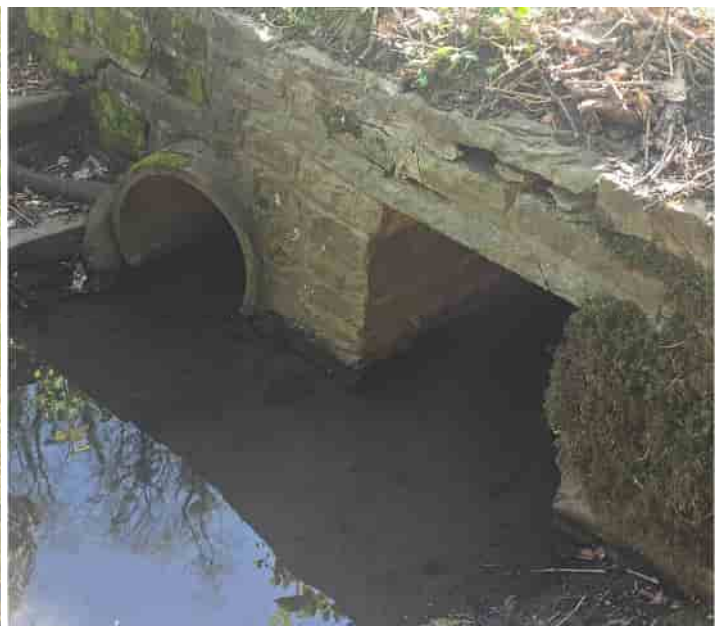
Location D – Culvert Outfall to Watercourse
