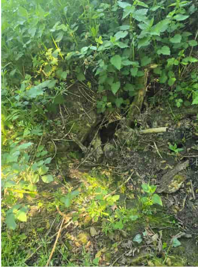
Location A - Culvert Crossing
