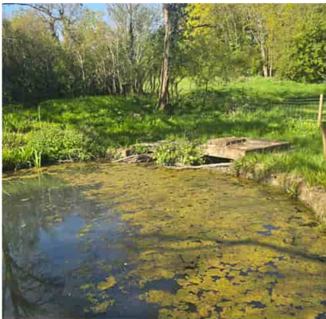
Location C – Pond Outfall to Culvert
