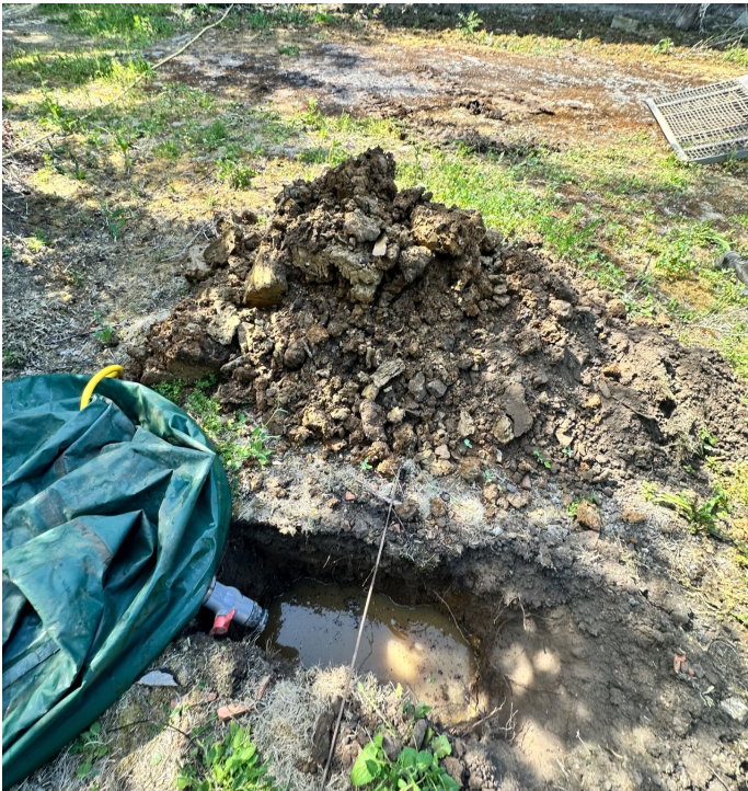
Trial Pit A – Pit A Photo
