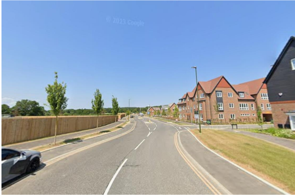
Figure 4: Moat Road, Horsham
