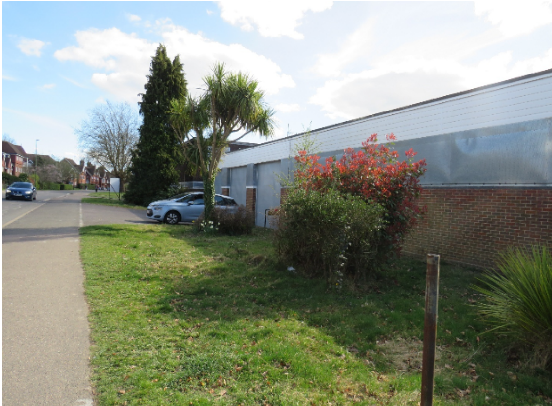
Picture 1; Looking southeast over the front of the site
