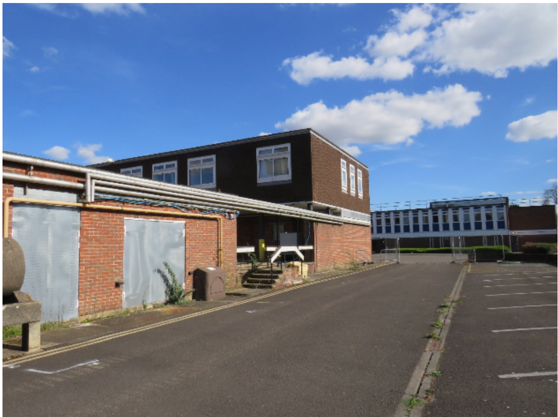
Picture 3; The rear of the site – old buildings and sealed surface.
