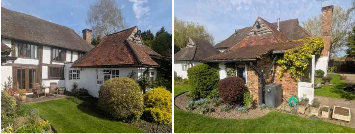
Figure 04 – Rear Elevation of Woodreeves showing existing single storey rear extensions
