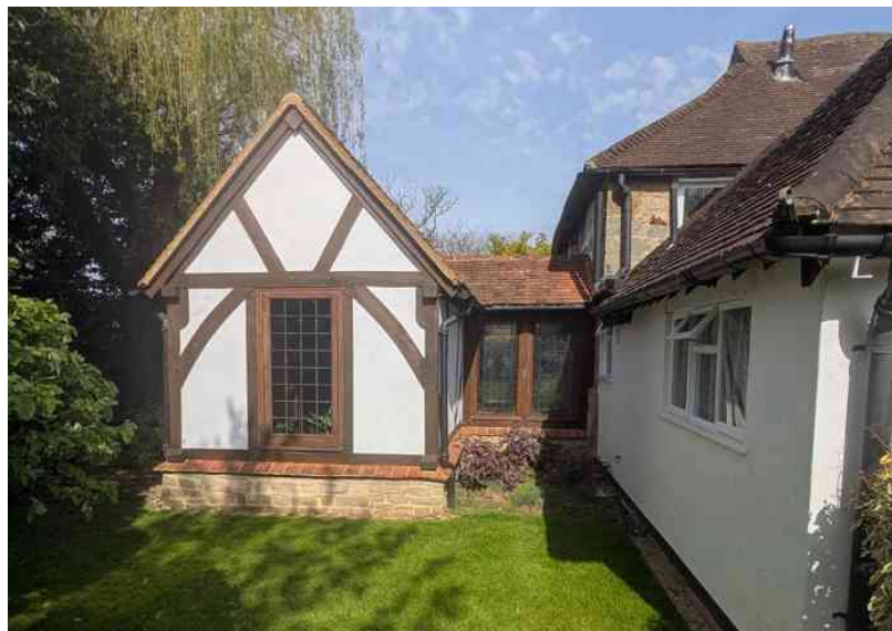
Figure 05 – Oak framed porch extension [Western Elevation] viewed from rear
