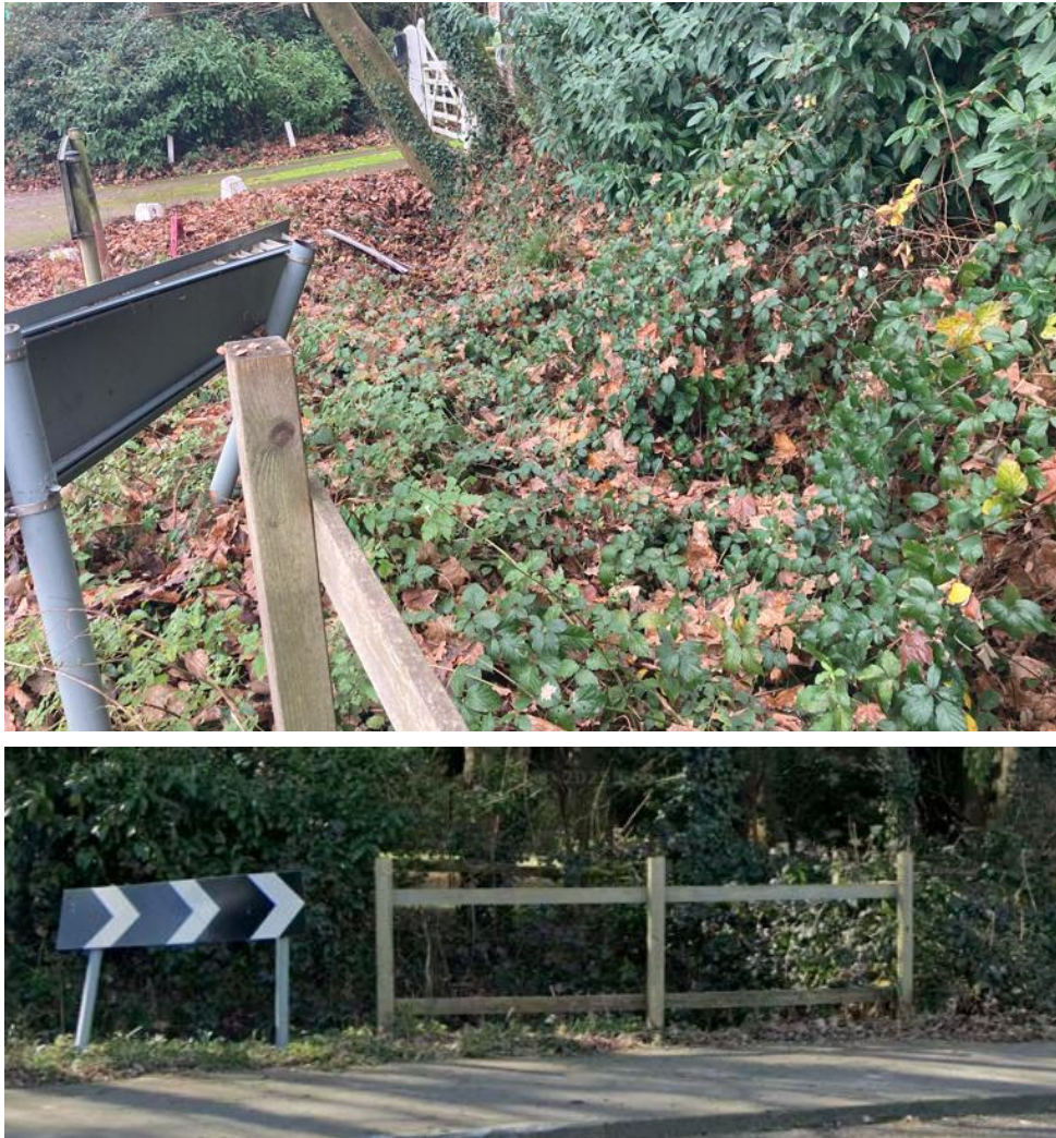
Figure 6.2 – Photographs of the existing ditch.
