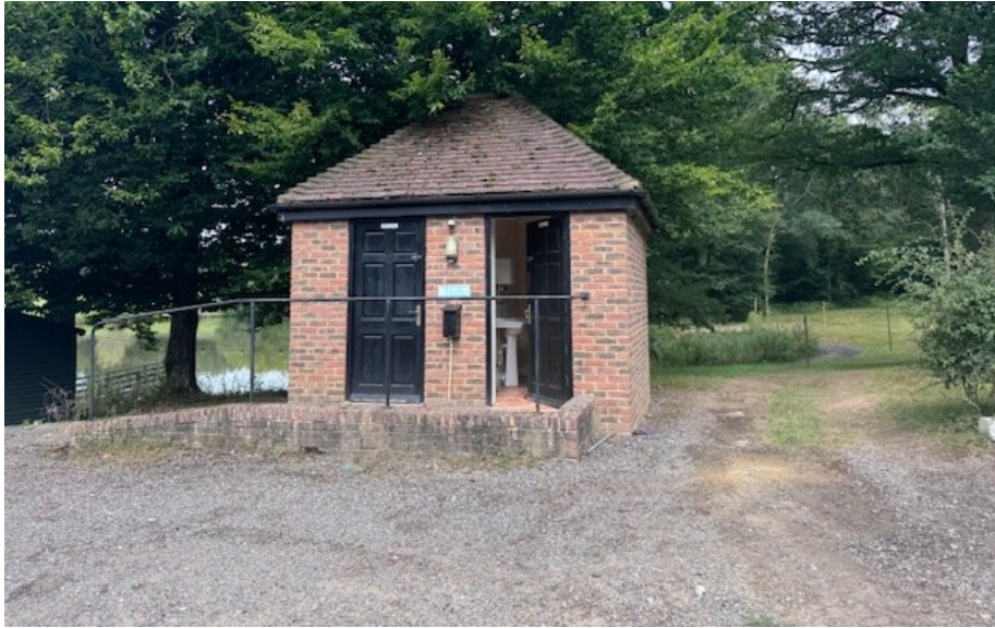
Figure 2.4 - WC Block and Facilities Building
