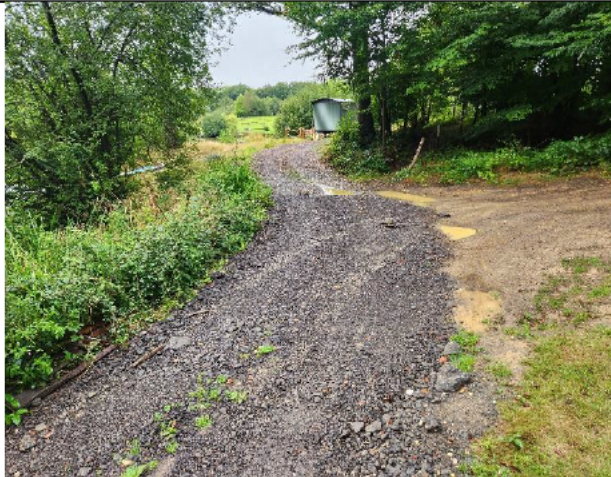
Photograph 1 – pre-existing gravel access track.
