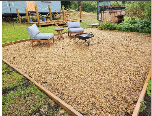
Photograph 4 – new shingle, decking, and hut mounted on a gravel bed.
