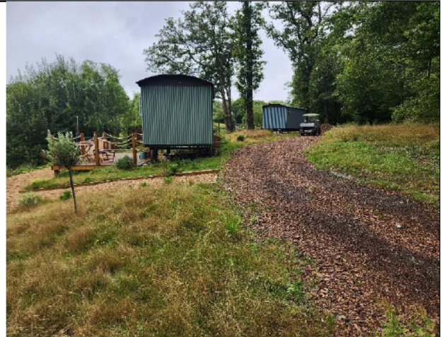
Photograph 2 – section of access track resurfaced with bark.
