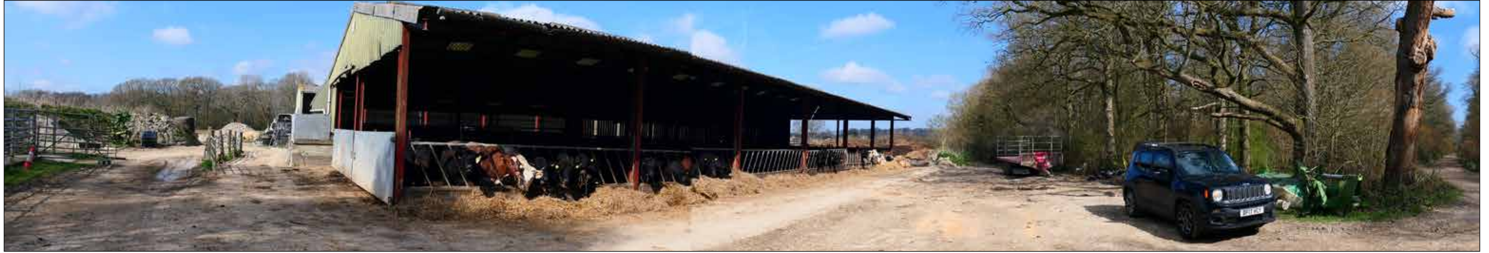
View j. Looking north towards the Site across the existing barns 27-03-25
