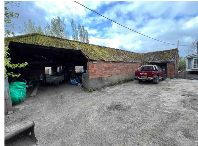
Existing Stables From North View
