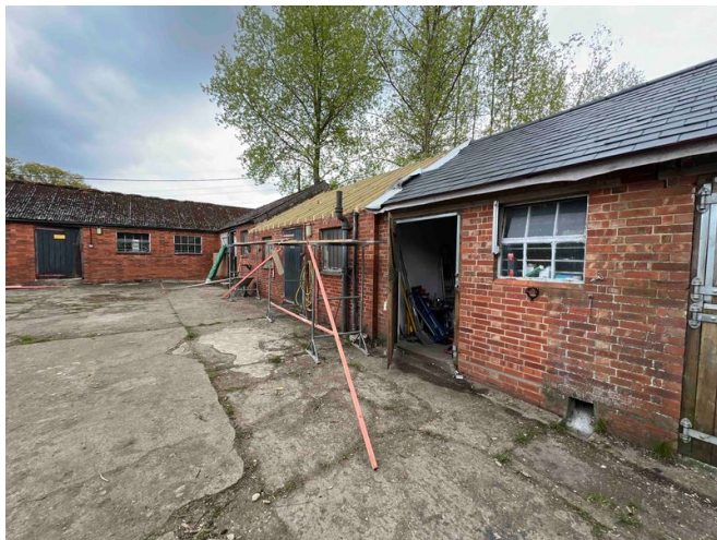
Existing Stables From Courtyard
