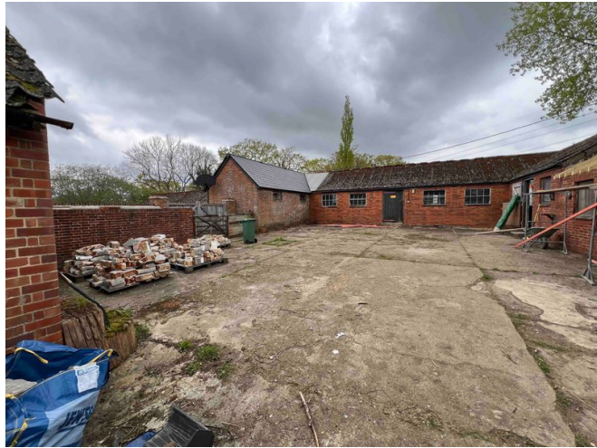
Existing Stables From Courtyard
