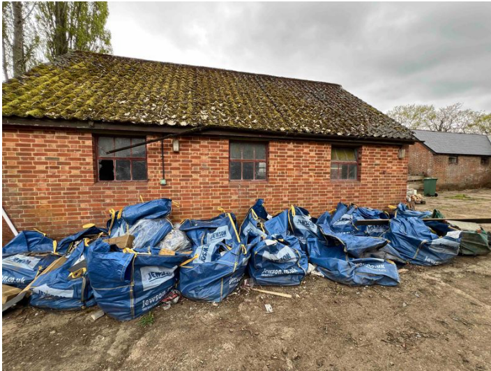
Existing Storage Barn
