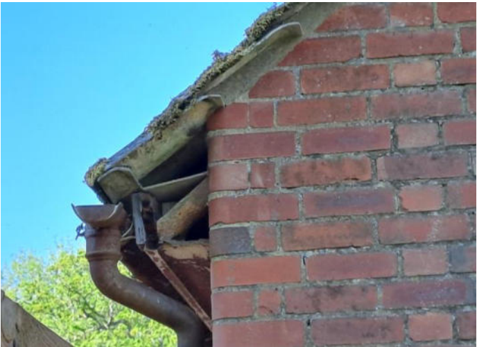
Photo 6: Displaying gap in soffit box in northeast corner of building B1.
