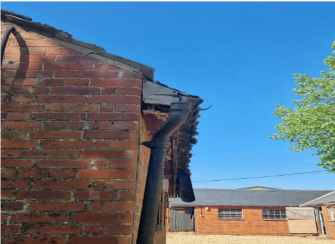
Photo 5: Displaying gap in soffit box in southeast corner of building B1.
