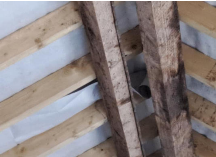
Photo 5: Displaying gap in soffit box in southeast corner of building B1.
