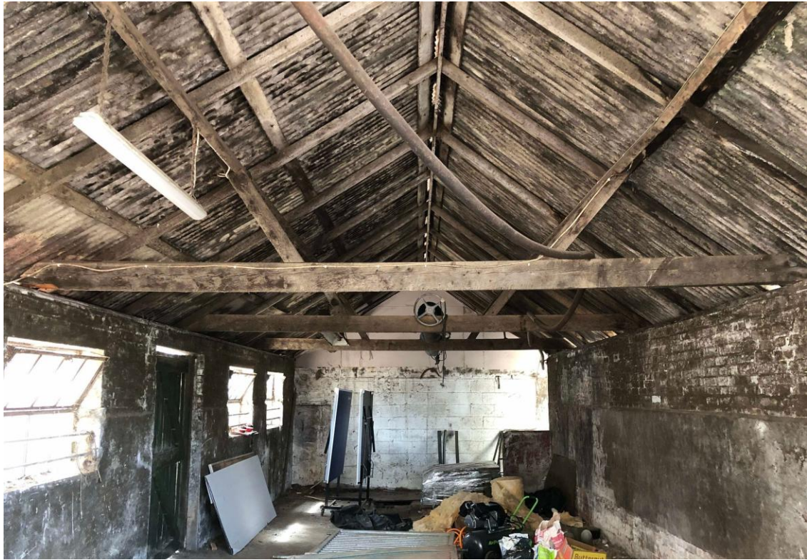
Fig 3: The oldest former farmstead outbuilding is that of the stable block range that sits to the north-east side of Lidford Farm House. The single storey range of buildings date from the 19 th Century and are currently disused.
