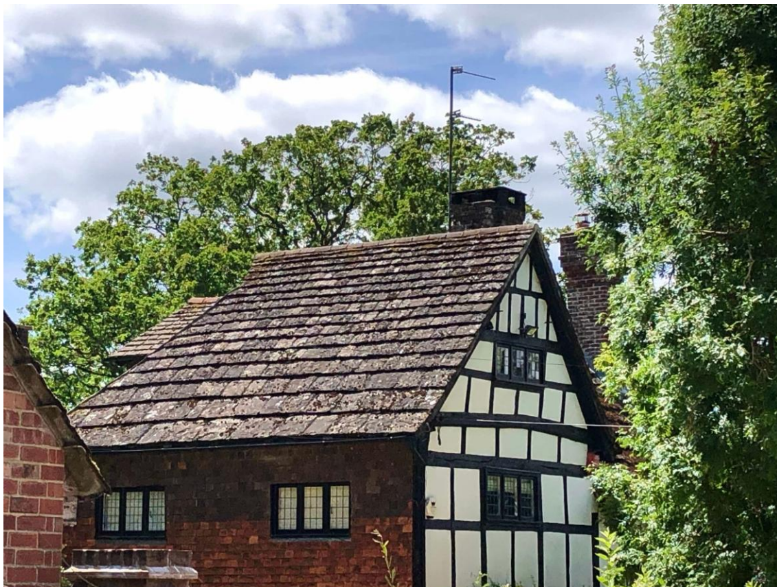
Fig 2: The proposed site sits adjacent to the Grade II listed building of Lidford Farm House and dates from the 16 th Century. It was the farmhouse for the former farmstead which included a historic range of buildings.
