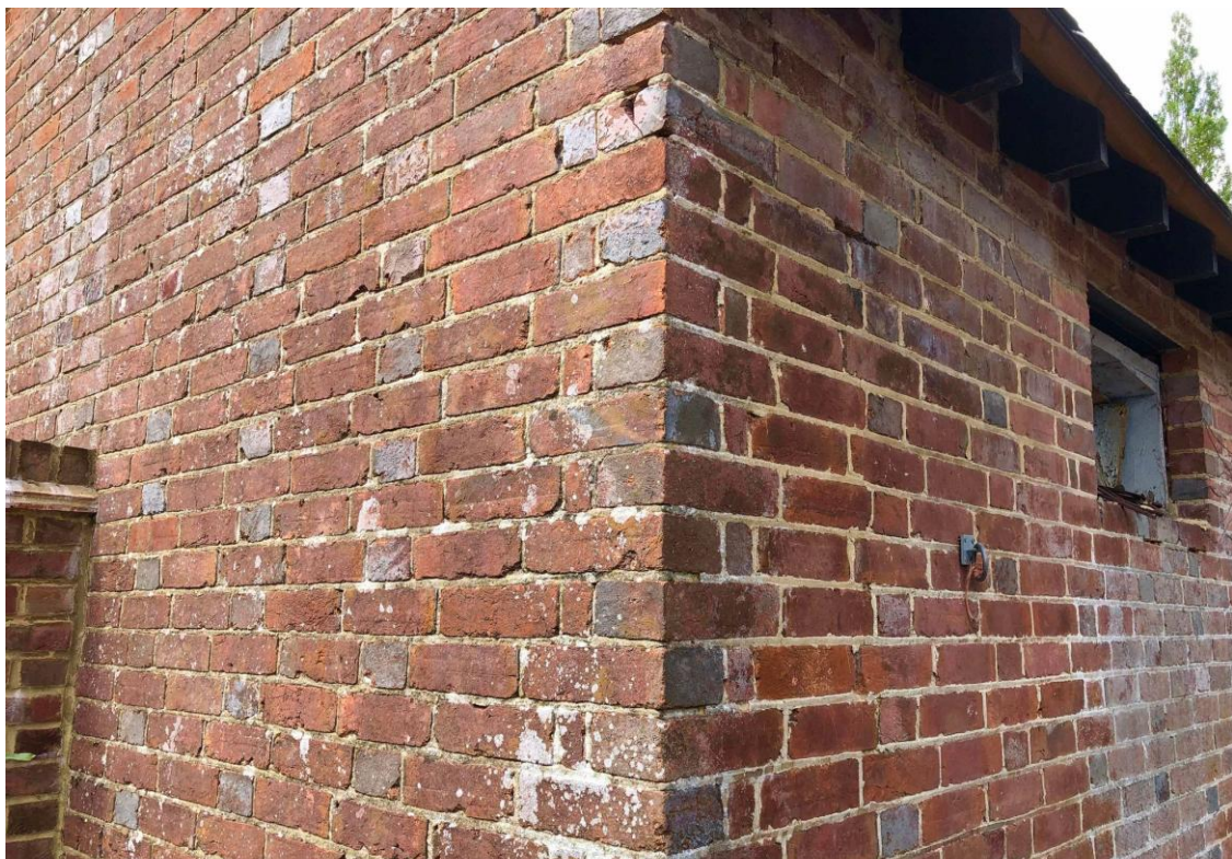
Fig 4: The former stable block now forms part of Taintfield Farm being separated across its western side. The historic outbuilding is brick built with grey headers and a slate roof with metal Crittall windows.
