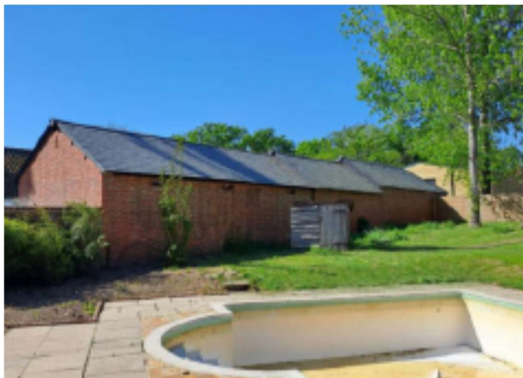
Figure 6: View of the barn from the eastern aspect
