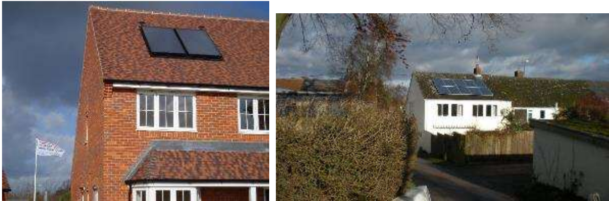
Figures 3 & 4: Solar thermal and solar PV installations on roofs
