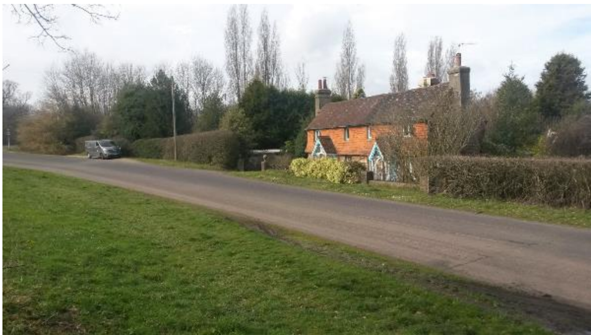
Plate 11: Moorhead farmstead, viewed towards the north-west
