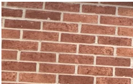
Existing face brick
