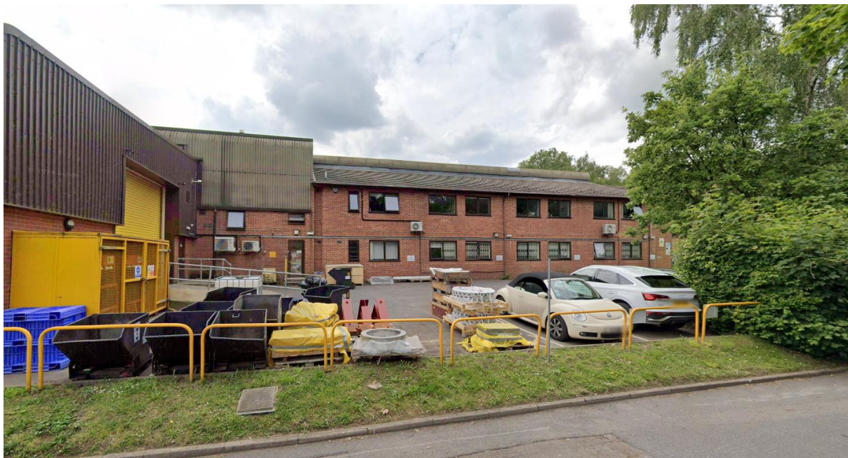
Photo 1 – Existing Condition – hardstanding and grass verge
