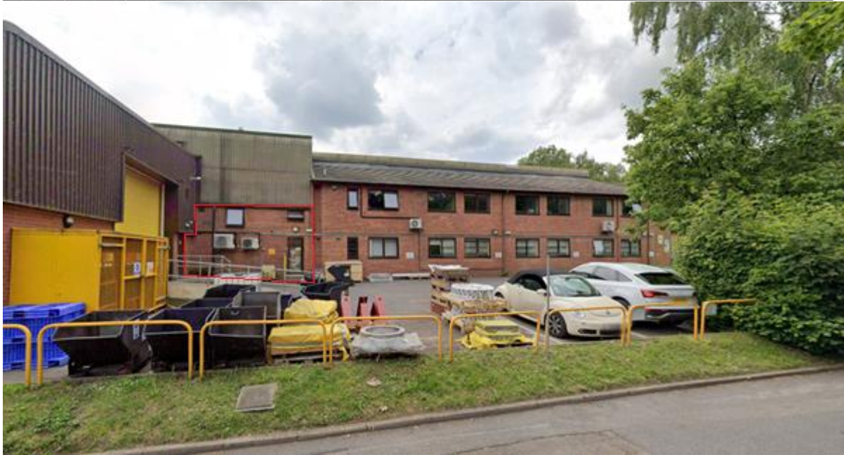
Photo 2 – Proposed location of extension – located on tarmacadam hardstanding.
