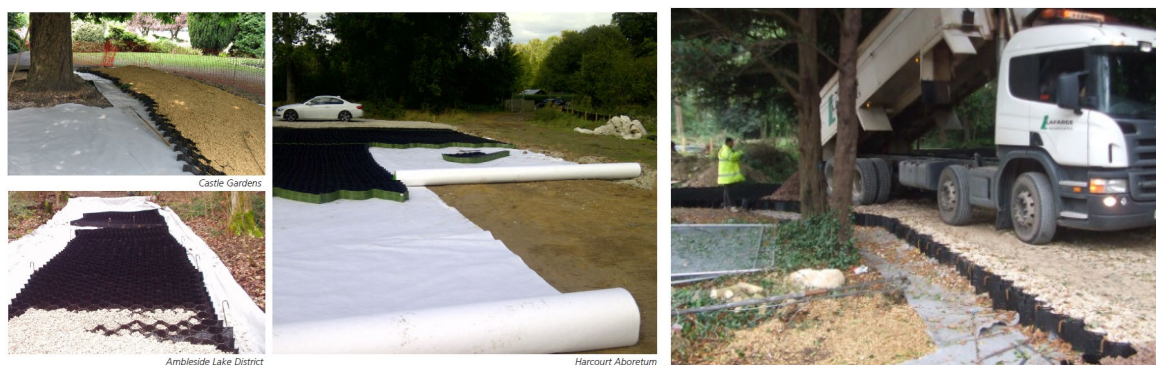
Figure 5: CellWeb® TRP depth variations and application.
