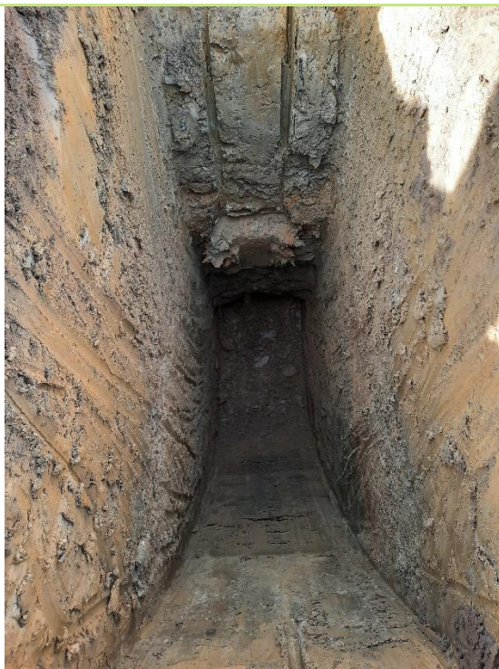
Plate 5 – Ground conditions encountered in TP10.
