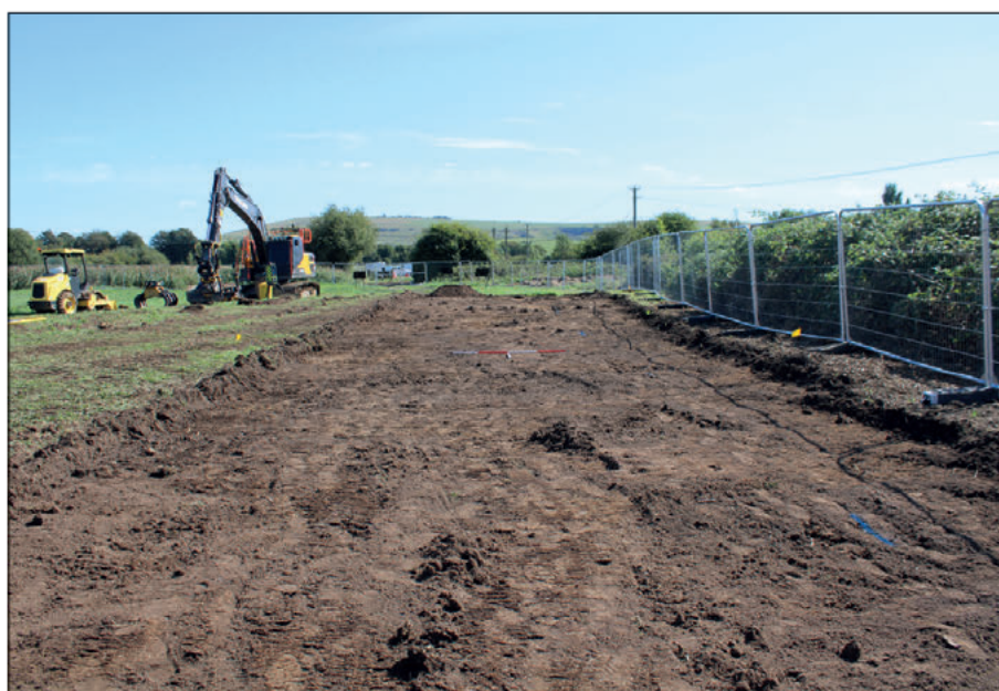
Figure 6: Trench 2, during excavation, 1 x 2 m and 1 x 1 m scale, looking west
