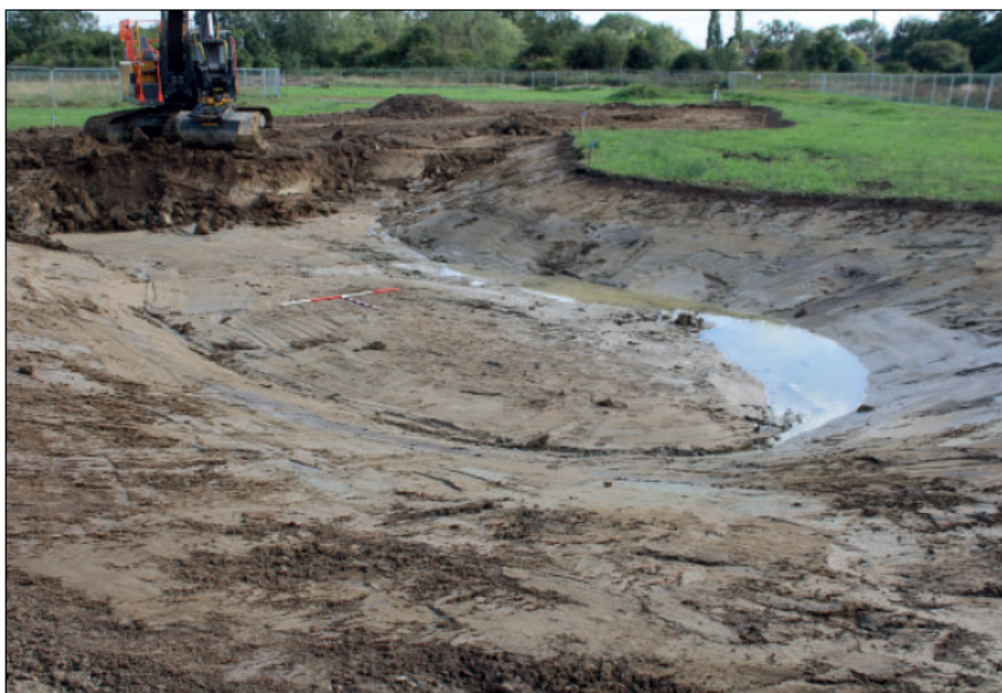
Figure 3: Trench 1, during excavation, 1 x 2 m and 1 x 1 m scale, looking north
