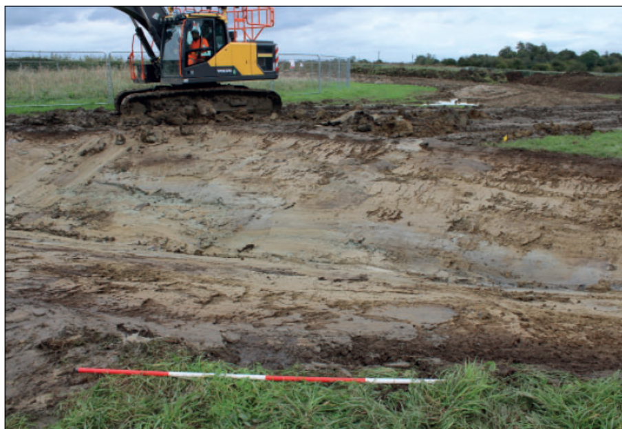
Figure 15: Trench 7, 1 x 2 m scale, looking east
